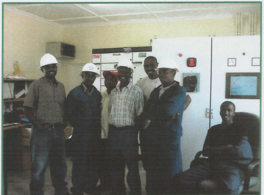
Oserian operators in the control room at the plant.
