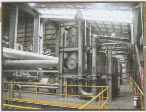
Vacuum system components provided by GDA included a Graham two-stage steam jet ejector, intercondenser, and aftercondenser for each 11 MW unit.
