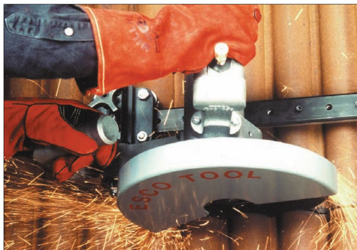
The PANELHOG® APS-438 Air Powered Saw glides along the EscoTrack System for boiler tube panel removal, producing a straight, clean horizontal cut that requires no further rework.
