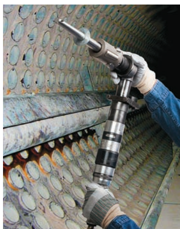
Available for sale or rental, tube expanding kits are custom fitted to meet your needs.
